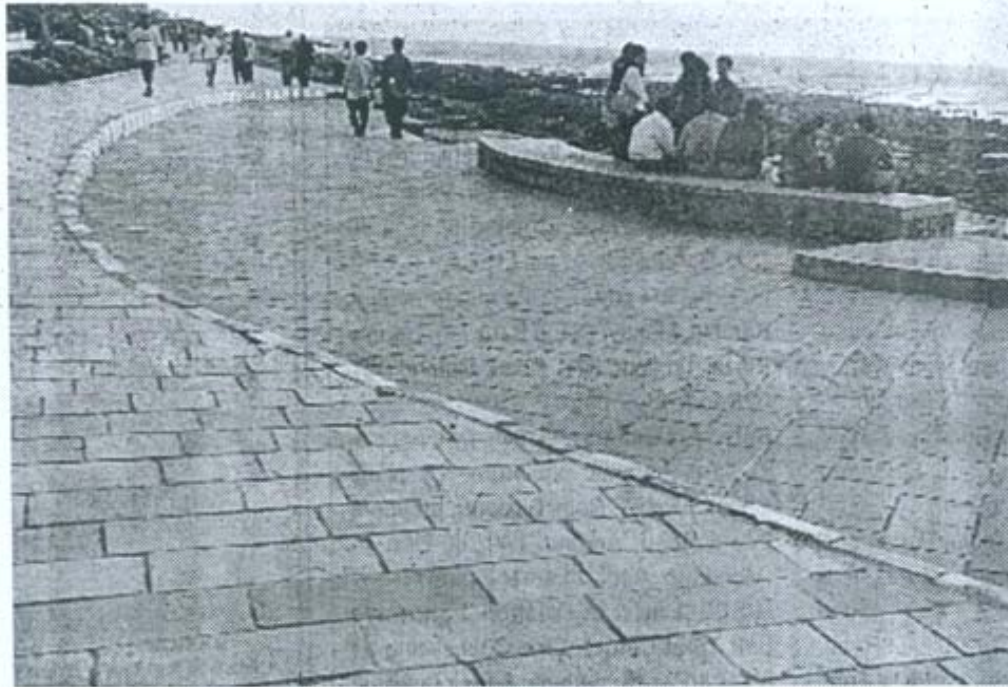
Bandra Bandstand after the redevelopment work
